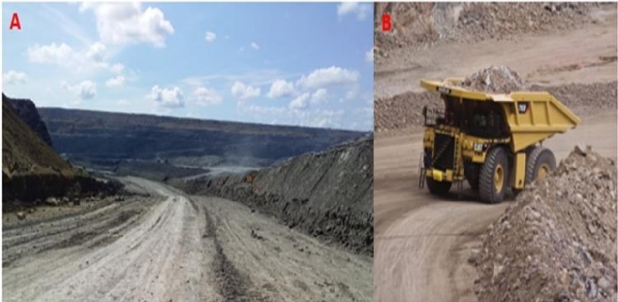
Figure 2. A. El Descanso mine roads. B. 793F mining trucks.
